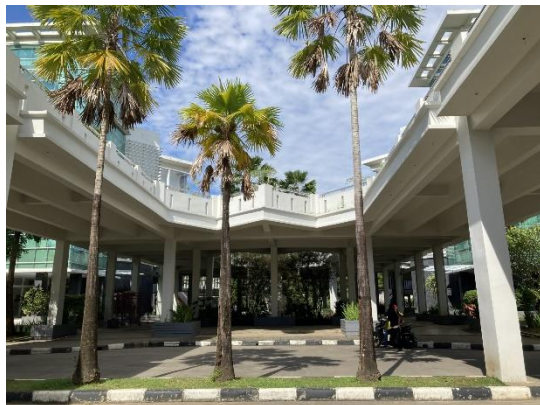
Photo 1: Pedestrian deck separating vehicles and pedestrians and connecting buildings (Source: Photographed by the evaluator)
