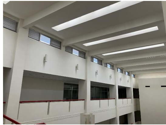
Photo 4: Environmentally friendly design with natural light streaming in from the ceiling (Source: Photographed by the evaluator)
