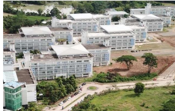
New campus of the FoE, UNHAS constructed under the project (Source: Project Completion Report)
