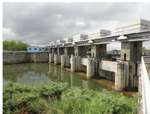
Song Luy Headworks (Source: External evaluator)
