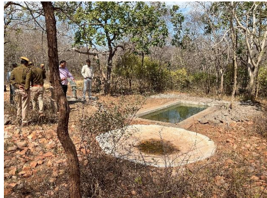
Photo 5: Fence installed around the wildlife sanctuary to prevent livestock intrusion. Photo 6: The water drinking basins for animals. The shallow, bowl-shaped design prevents small animals from falling into the water. (Photos by the external evaluator).
