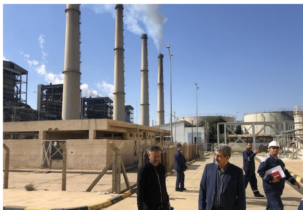
Image 1: Al-Mussaib Thermal Power Plant. The boilers for Units 1 to 4 are on the left. (source: Photographed by field survey assistants)
