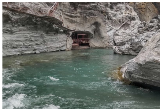
Photo 8 A simple water intake installed as an emergency measure
