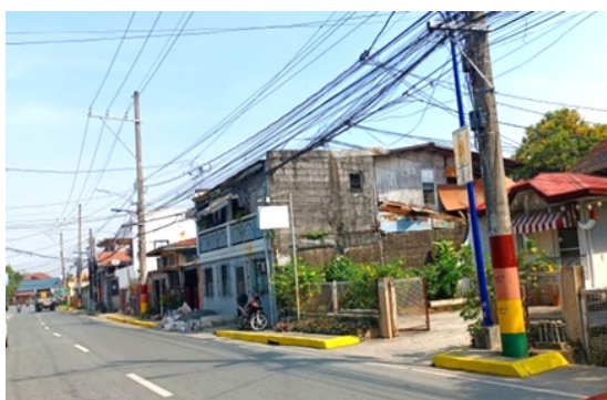
Photo 3: The Utility Pole is Utilized to Indicate the Water Level Danger (Imus River Sub-Project)
