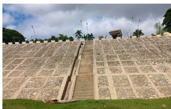
Photo 4: Revetment Developed Along the Cagayan River (Cagayan River Sub-Project)
