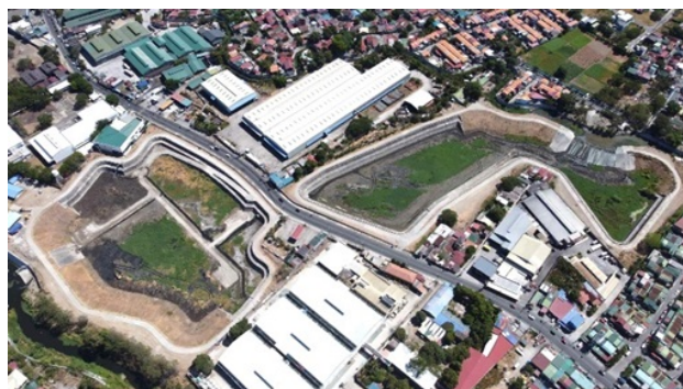
Retarding Basin Developed Under the Imus Sub-project (Source: DPWH)
