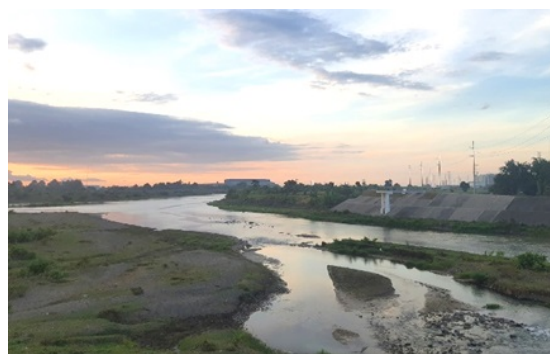
Photo 2: Revetment Constructed as Part of the Tagoloan River Sub-Project
