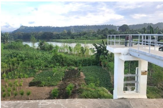
Photo 5: Developed Sluice Gate and Farmland (Field) (Tagoloan Sub-Project)
