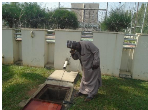
1. Staff of FCTWB using the Leakage Detection tool
