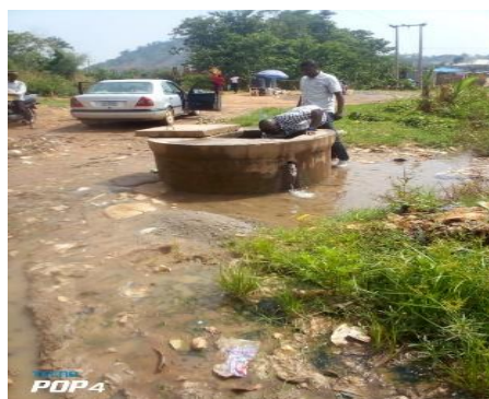
4. Second location of detected leakage in Apo district.
