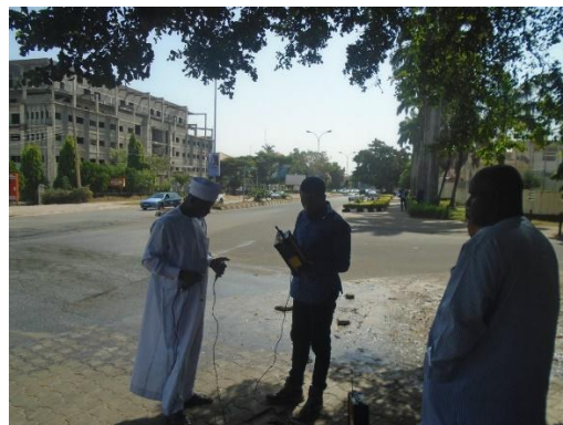
2. Leakage Detection tool Calibration in progress
