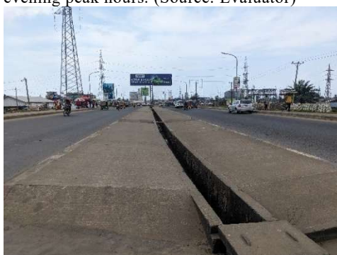
Photo 11: Well-maintained drainage ditches at the median of the road by the industrial area (Source: Evaluator)
