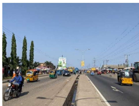
Photo 2: Near the 2km point at the time of the ex-post evaluation (April 2025) (Source: Evaluator)
