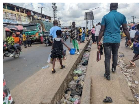
Photo 12: The issue of illegal waste disposal is particularly severe in the area around the Red Light Market. (Source: Evaluator)
