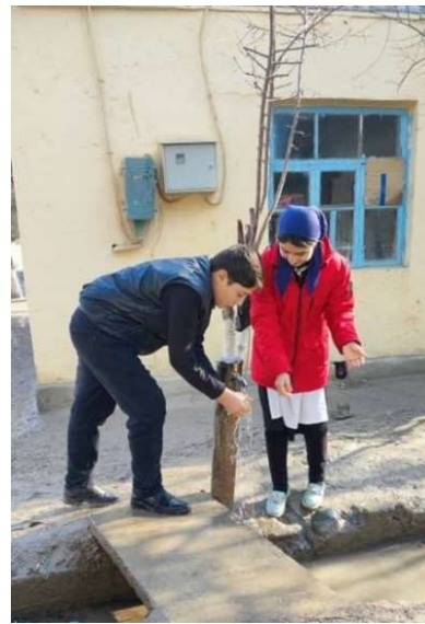
Photo 2 Water tap installed at school (Photo taken by the local consultant)
