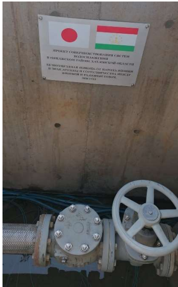
Photo 1 Intake well (Photo taken by the local consultant)
