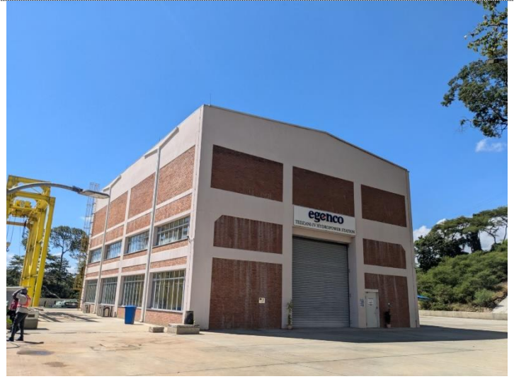
Photo 2. Tedzani Hydropower Plant Unit IV Powerhouse (Source: Taken by the External Evaluator)
