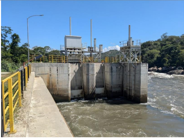
Photo 1. Intake of Tedzani Hydropower Plant Unit IV (Source: Taken by the External Evaluator)
