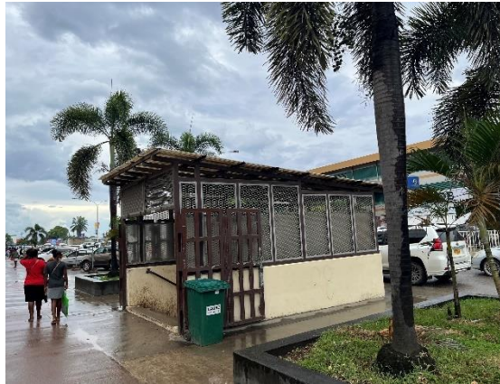
Photo 9: Renovated and reused underpass (Photo 1) (Source: Photo taken by the external evaluator)
