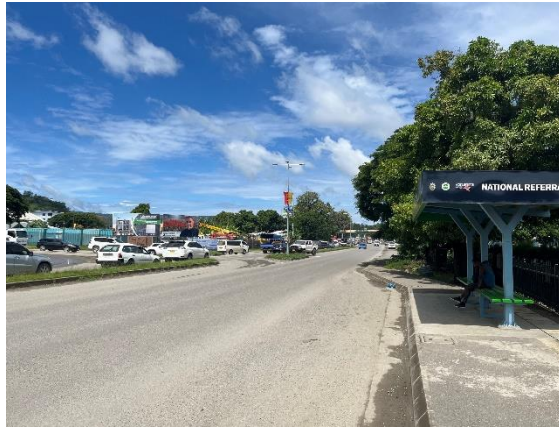
Photo 1: Upgraded Kukum Highway and installed bus bay (Source: Photo taken by the external evaluator)
