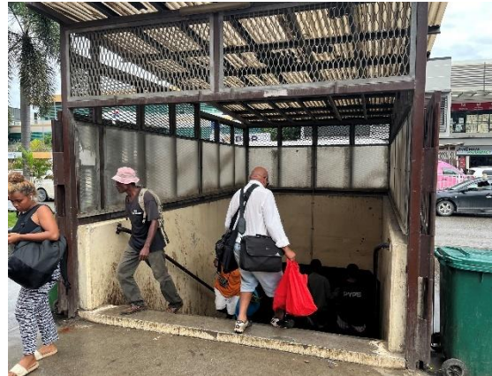
Photo 10: Renovated and reused underpass (Photo 2) (Source: Photo taken by the external evaluator)
