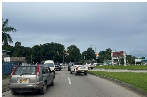
Upgraded road and improved roundabout (Source: Photo taken by the external evaluator)
