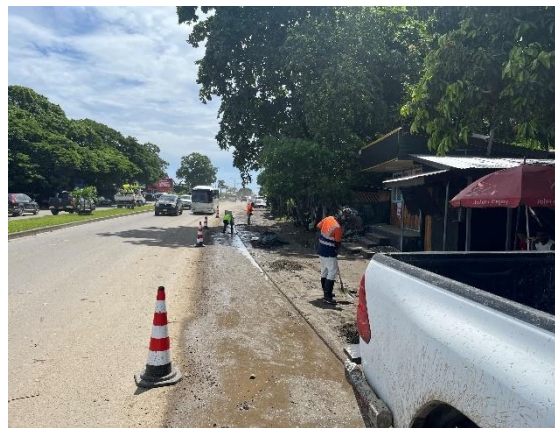
Photo 8: MID contractor cleaning the roadside ditches
