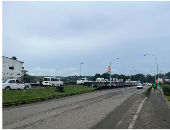
Photo 2: Widened New Mataniko Bridge (the lane on the far side is the widened two lanes) (Source: Photo taken by the external evaluator)
