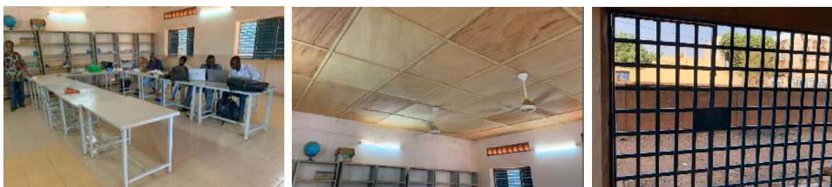
Photo 6 (Left): View of the staff room (A-04: Tampouy E, F)
