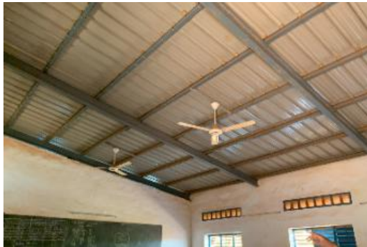
Photo 1 (Left): Corrugated metal roof of a classroom (A04: Tampouy E, F)
