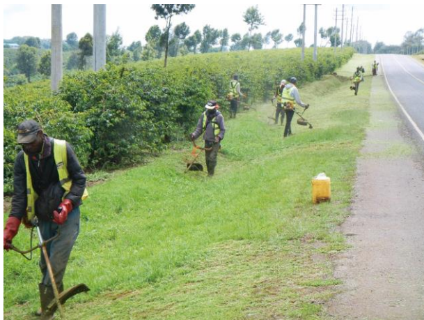
Maintenance of roadside grass through PBC (Photo taken by JICA expert)
