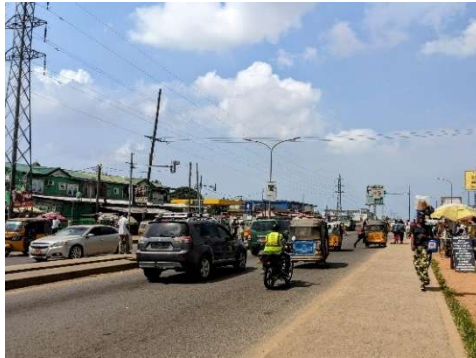
Photo 7: New Georgia Junction. Traffic signals are functioning. Traffic flow is smooth even in peak hours. (Source: Evaluator)
