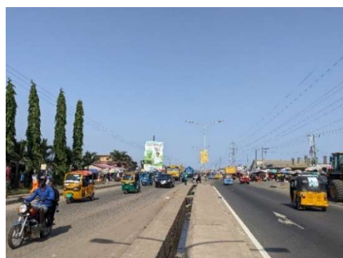
Photo 2: Near the 2km point at the time of the ex-post evaluation (April 2025) (Source: Evaluator)
