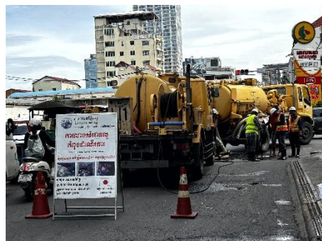
Photo 2: DSO officers cleaning pipes with sign board) (taken by evaluator)
