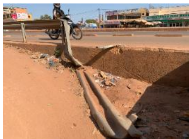
Photo 5: Damaged Guardrail Photo 6: Pedestrian Bridge with Broken Tiles Photo 7: Damaged Bus Stop
