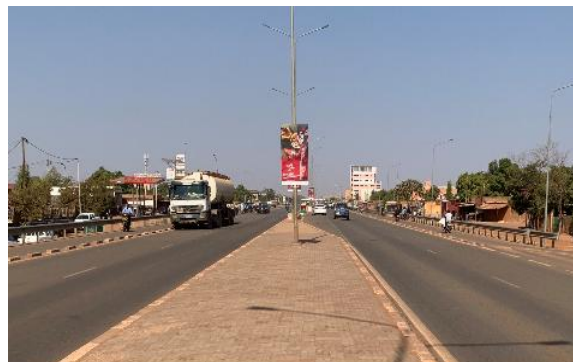
Rehabilitated Tansoba Bypass Road
