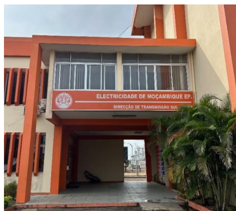
Photo 1 Infulene Substation (source: taken by the external evaluator)
