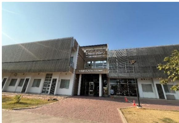
New Building of Setthathirath Hospital Constructed by the Project (Photo taken by the external evaluator) 2
