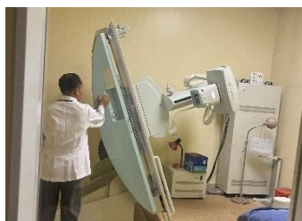
Photo 1. X-ray Fluoroscopy Unit Installed at Setthathirath Hospital
