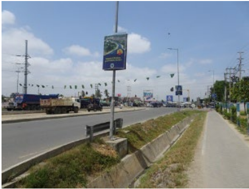
Photo 1. New Bagamoyo Road (source: Evaluator)
