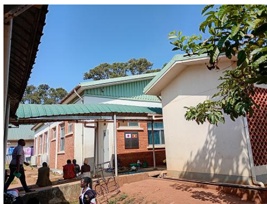
Photo 5: The Delivery Suite Constructed at Lira RRH. In the Foreground is the Generator Room (source: taken by the evaluator)
