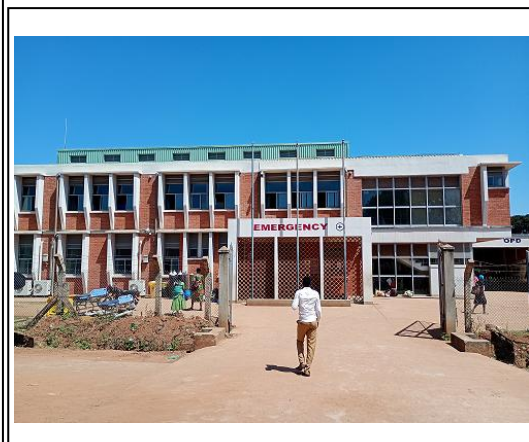
Photo 1: OPD/Casualty Block at Lira RRH Built by the Project (source: taken by the evaluator)
