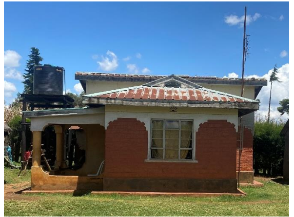
Improved housing and water tank owned by a farmer who applied SHEP Approach
