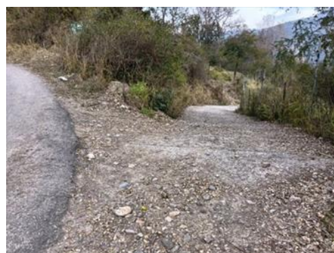
Photo 4: Farm access road leading to the CCA in Hamirpur District. The total length of the improved road is 596 meters. (Source: Photo taken by Evaluator)
