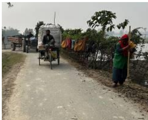
Photo 2: Improved rural road (Rangpur District) (Source: Taken by the evaluator)
