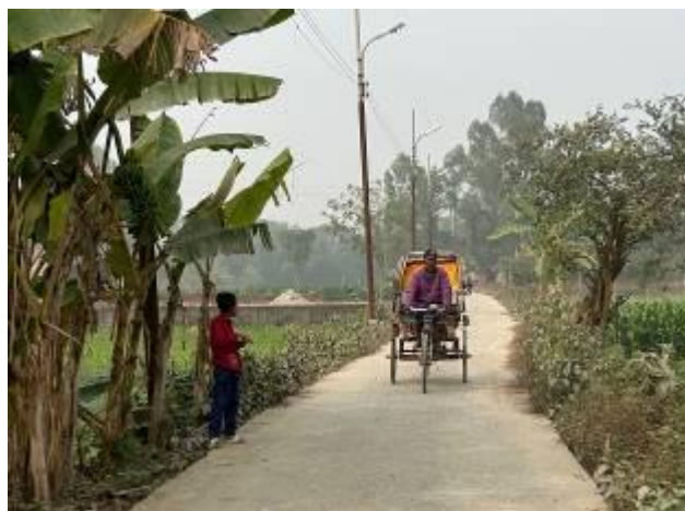
Photo 1: Urban road and streetlights developed under the project in Rangpur District (Source: taken by the evaluator)
