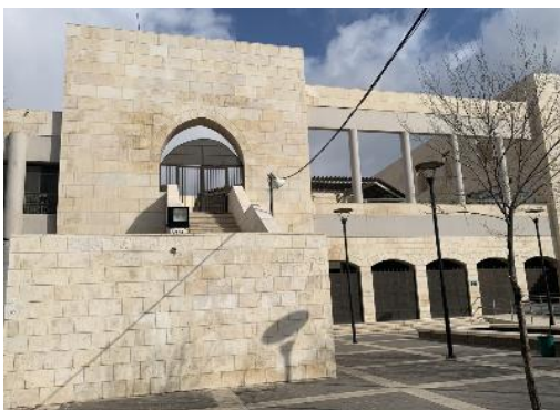
One of the sites under Programme No. 6 (Ragadan Bus Terminal in Amman) —Repair of stone walls (Source: Taken by the evaluator)
