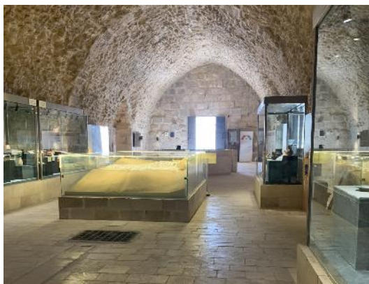
One of the sites under Programme No. 6 (Karak Museum) —Repair of flooring (Source: Taken by the evaluator)
