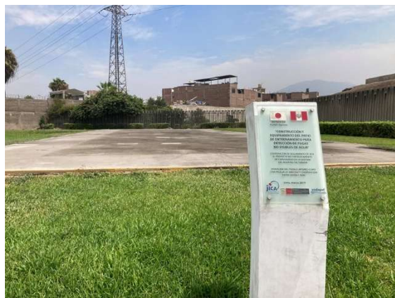
Photo 6. Leak detection training yard 9
