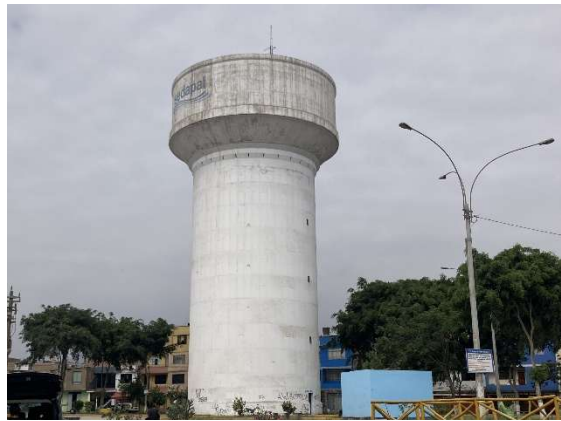
Rehabilitated Distribution Reservoir 2
