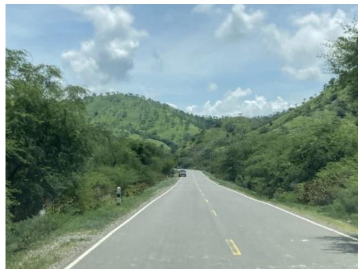
Condition of the Improved National Road No. 1 (Source: Taken by the evaluator)
