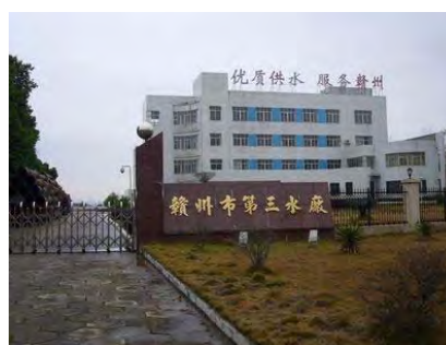
Ganzhou No. 3 Water Treatment Plant
