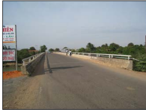
Photo 7: Luy river bridge
