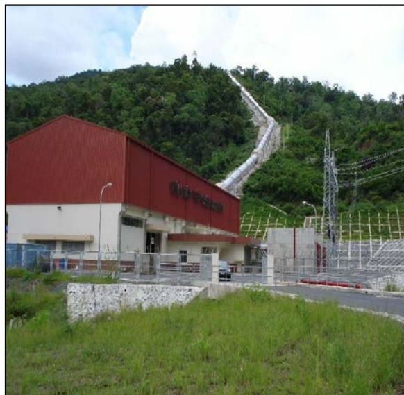
Dai Ninh Power house
