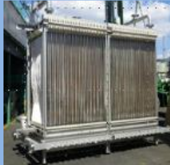
Submerged membrane filtration technology (Optimal for treatment of seasonally varying highly turbid surface water)
