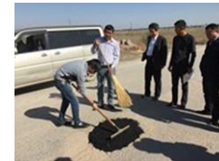
Patching Excel in a pothole
