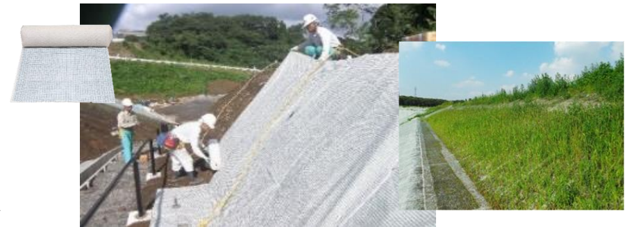
Erosion prevention vegetation sheet (Quilket)
