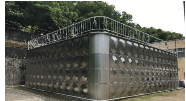
Proposed product "Stainless Steel Clean Water Reservoirs Saitama Prefecture, Japan(1,000m 3 )
