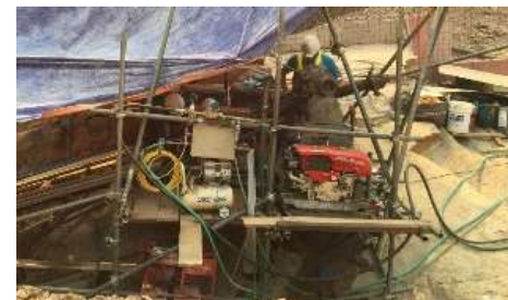
Drilling in dam site(angled)
