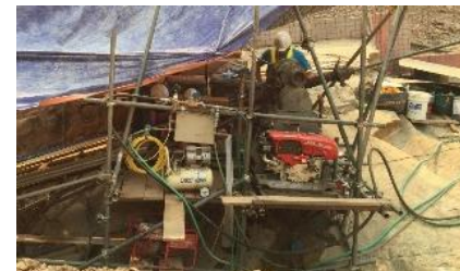
Drilling in dam site(angled)
