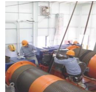
Maintenance for the main device of a crane
