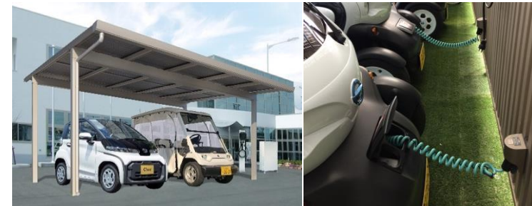
AOZORA Outlet (Solar carport with battery storage and charging function)
