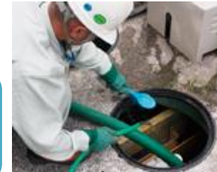
Cleaning of a septic tank
