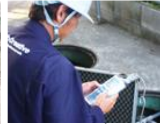
Monitoring for treated wastewater
