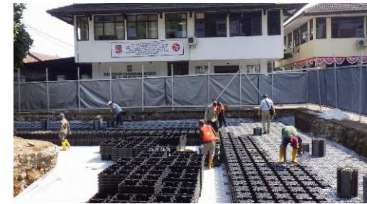
Construction example of PRSS
