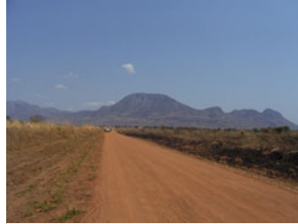
The present conditions of the road which will be build by the project
