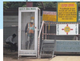
Safety measures for civil works
