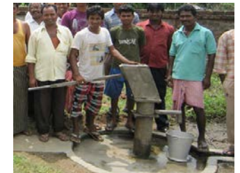
The well for current water supply
