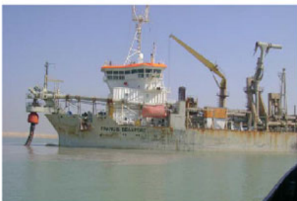
Dredging (Completed in March, 2011)
